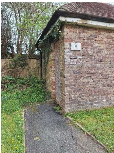
Former Gents (Derelict)
