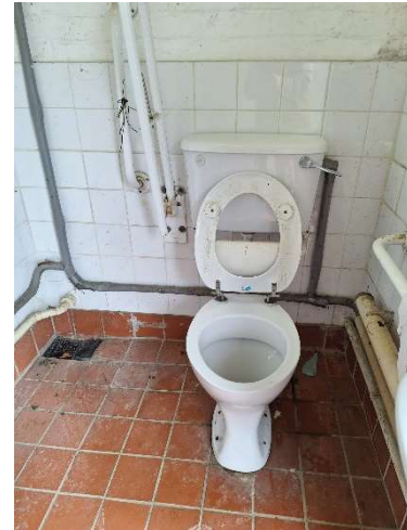
Interior of Unisex WC
